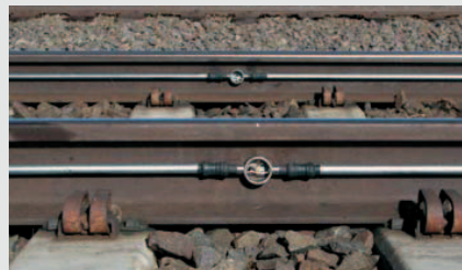
Picture 3: Rail with installed sensor
